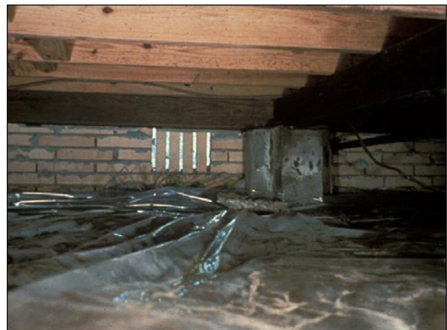
*Polyethylene is widely used as a crawl space ground cover.*
