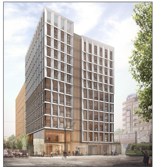
Architectural rendering of Framework, a 12-story CLT building project in Portland, Oregon.
