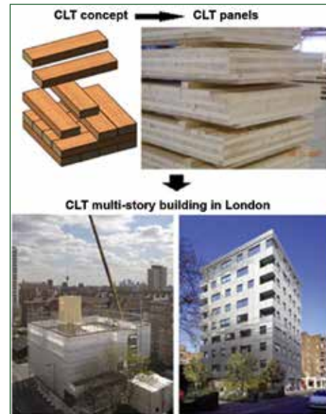
Figure 1—CLT concept and use in a nine-story mid-rise building in London.
