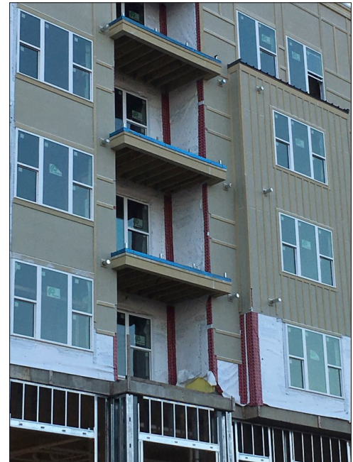
Construction in Charlotte, North Carolina. (Photo credit: Home Innovation Research Labs)
