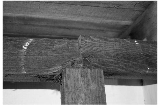
Figure 2. Crushing failure on a salt-damaged joist in the bilge of the *Eureka*.
