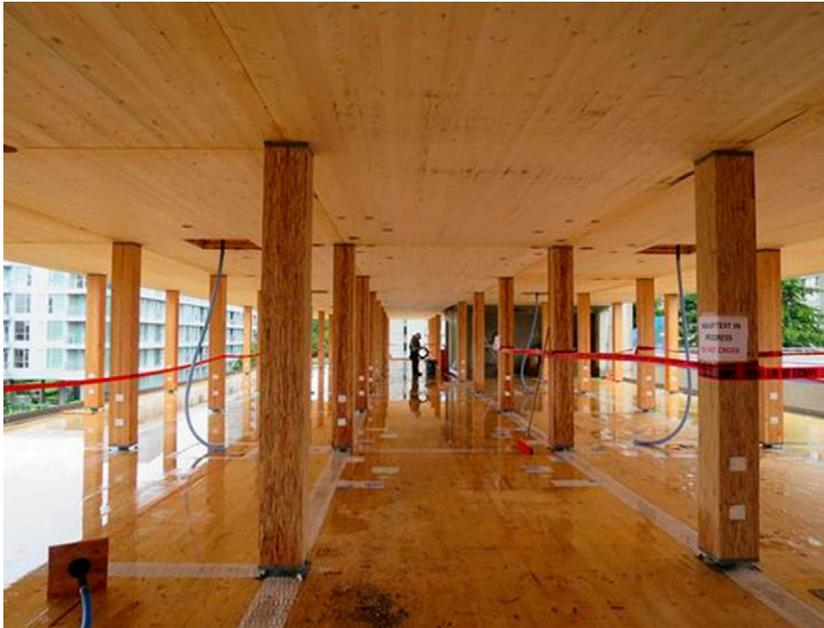
Figure 3. Water accumulating on a cross-laminated timber floor following a rainstorm.
