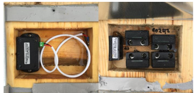
Figure 3: Sensors located in pockets notched in CLT panels
