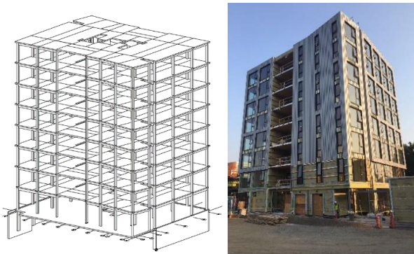
Figure 1: Eight-story mass timber building structural schematic and photograph during construction
