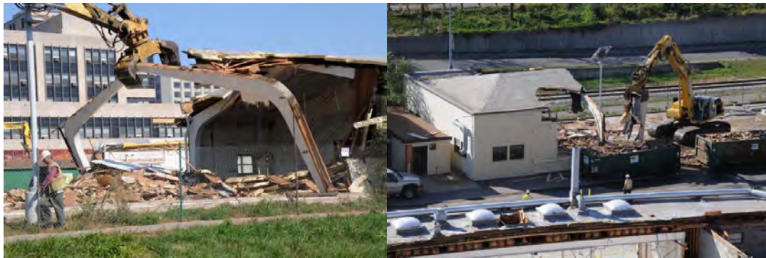
Figure 2 —Deconstruction of FPL’s glued-laminated arch building in 2010.
