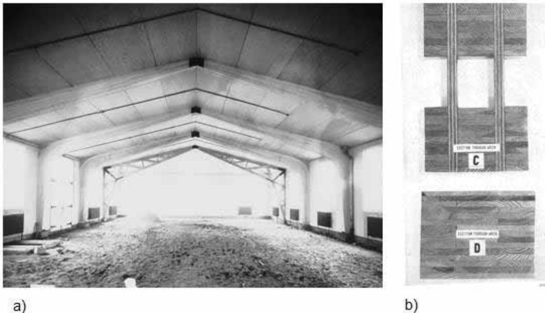
**Figure 1**—a) Inside view of the USDA Forest Products Laboratory service building, b) Cross-section views of C-type and D-type glulam used as the bearing structural components in the building.
