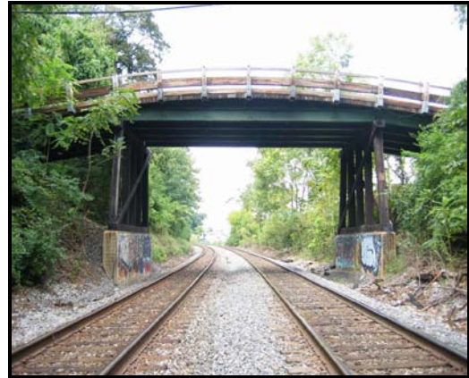
Figure 1 – View of East Deer Park Drive Bridge.
