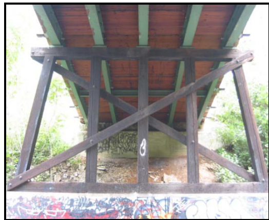
Figure 2 – Timber column-bent support pier.
