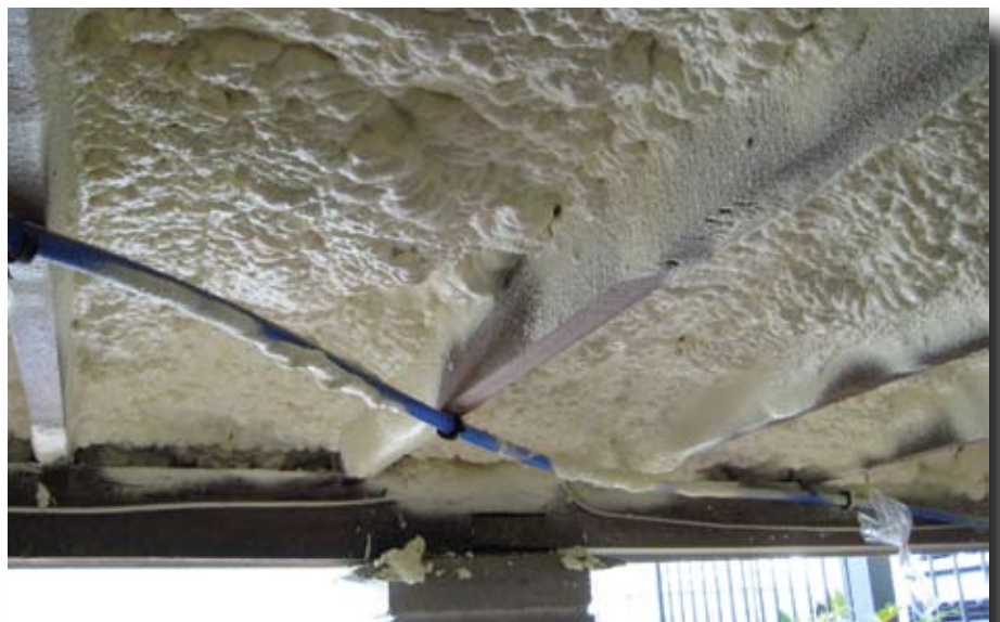
Figure 4c. Example of open cell spray foam.
