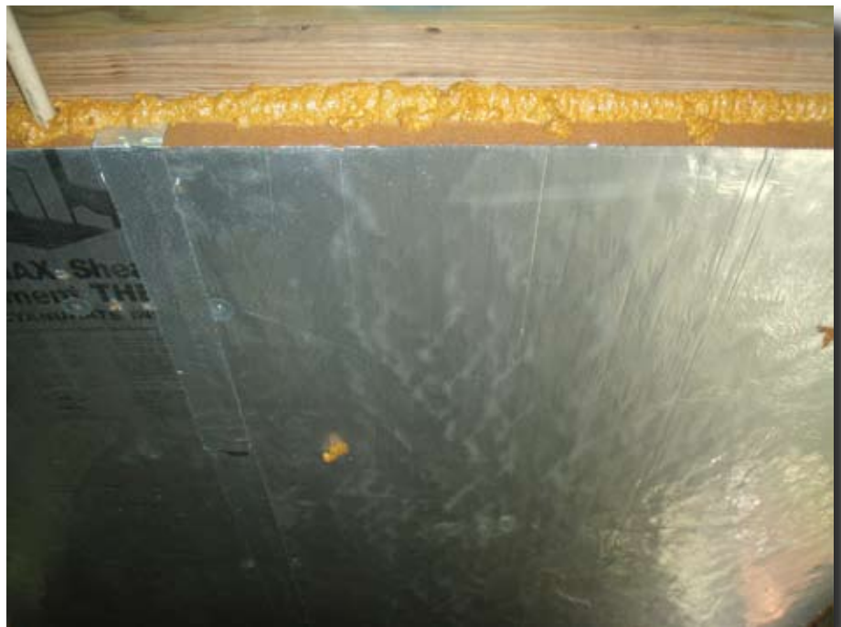
Figure 4a. Example of rigid, foil-faced polyisocyanurate foam.
