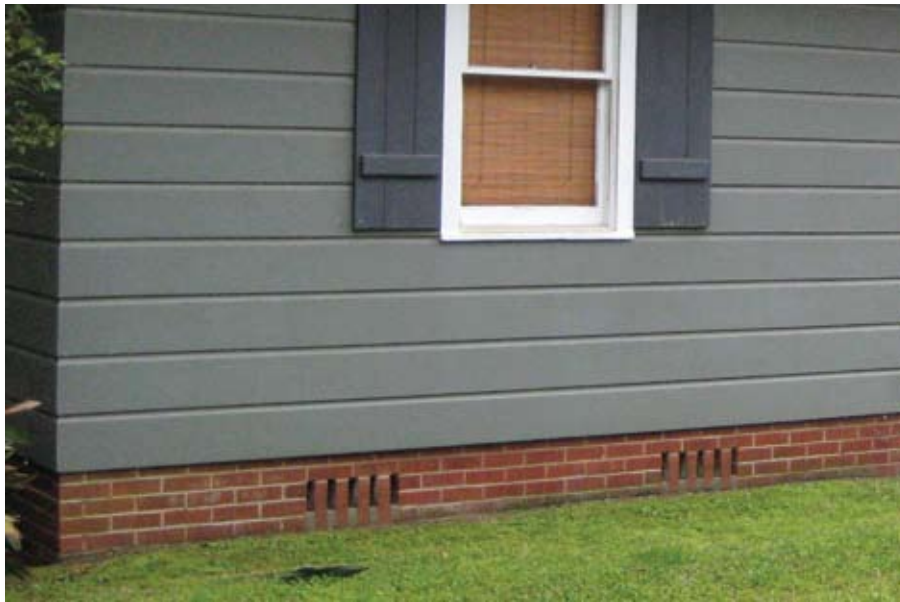
Figure 2. Example of a wall-vented crawl space.
