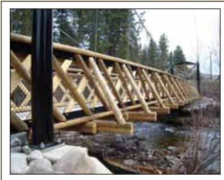
The Rattlesnake Creek bridge near Missoula, Montana, was built using 6-inch-diameter lodgepole pine from a forest in Idaho to demonstrate the effective use of trees killed by the pine bark beetle.
