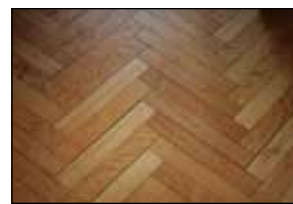
Several combinations of wood species were designed and laid out as test flooring on the FPL's fourth floor to measure effects of humidity, temperature change, and general use.
