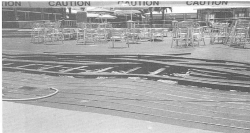
**Figure 9.** Warping due to thermal expansion of a plastic lumber deck in The Bahamas
