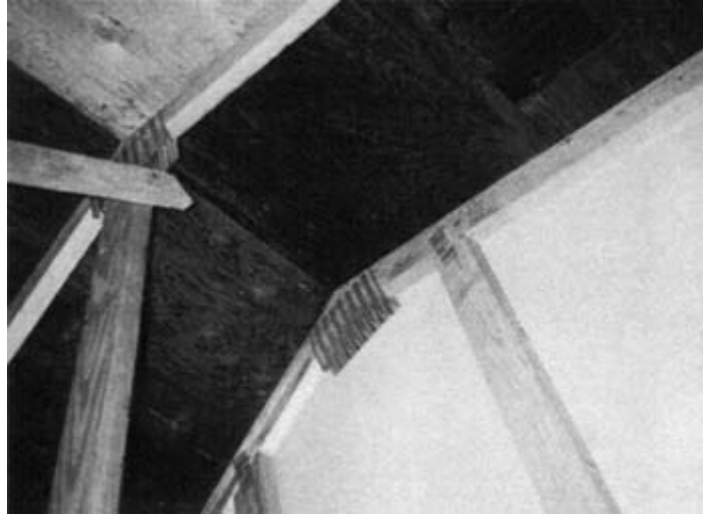
FIGURE 11.26 Example of fully serviceable untreated plywood roof sheathing (top left) adjacent to thermally degraded FR-treated plywood sheathing (center) used next to a gypsum-sheathed 60-minute-rated fire wall (lower right).
