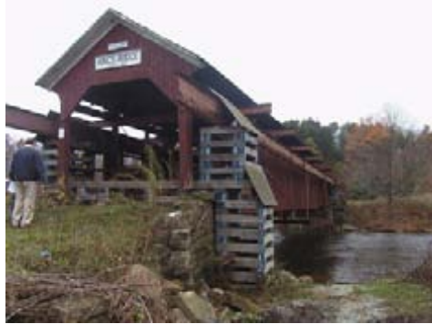
Figure 1 – Kings Bridge eastern portal w/ temporary truss system
