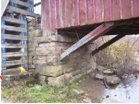
Figure 4 – Northern face of eastern abutment. (Note the separation of the wingwall face resulting from the horizontal thrust of the truss/arches after lower chords failed.)
