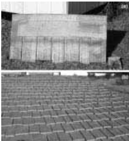
Figure 1. — Wood-thermoplastic composite roofing for Wisconsin exposure in 2001: (a) roof tile, (b) installed WTPC shingles.
