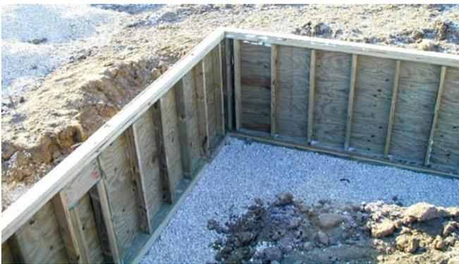
**Figure 1** CCA is still registered for some residential applications, such as permanent wood foundations.
