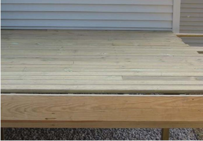
**Figure 5** CCA-treated supports and CBA-A treated decking.
