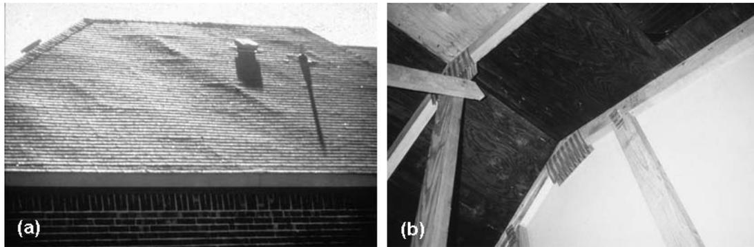
**Figure 1. a) outside view of failed FR-treated plywood roof sheathing; and b) top left—inside view of fully serviceable untreated plywood roof sheathing; center—thermally degraded FR-treated plywood roof sheathing; and lower right—gypsum-sheathed 60-minute-rated fire wall.**
