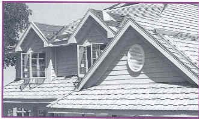
Figure 5. - Roof shingles made from natural fibers and thermoplastic on the demonstration house at the Advanced Housing Research Center, Forest Products Laboratory, USDA Forest Service, Madison, Wisconsin.
