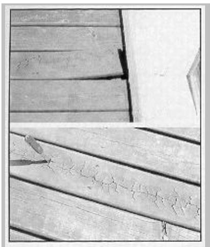
Figure 8—Warping (top) and excessive surface degradation (bottom) resulting from juvenile wood.
