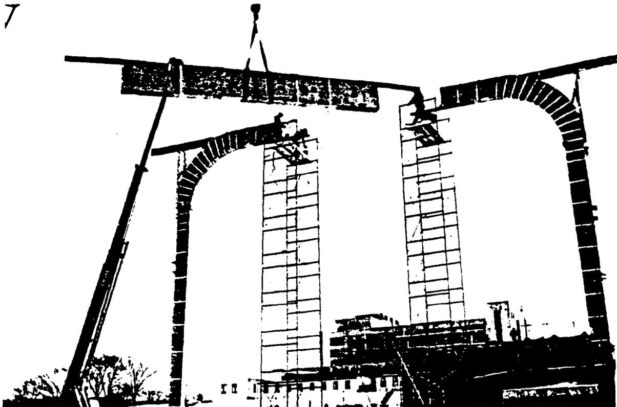
*Figure 8. Kraft paper covering these glued-laminated timber arches protects their surfaces during transport and erection.*
