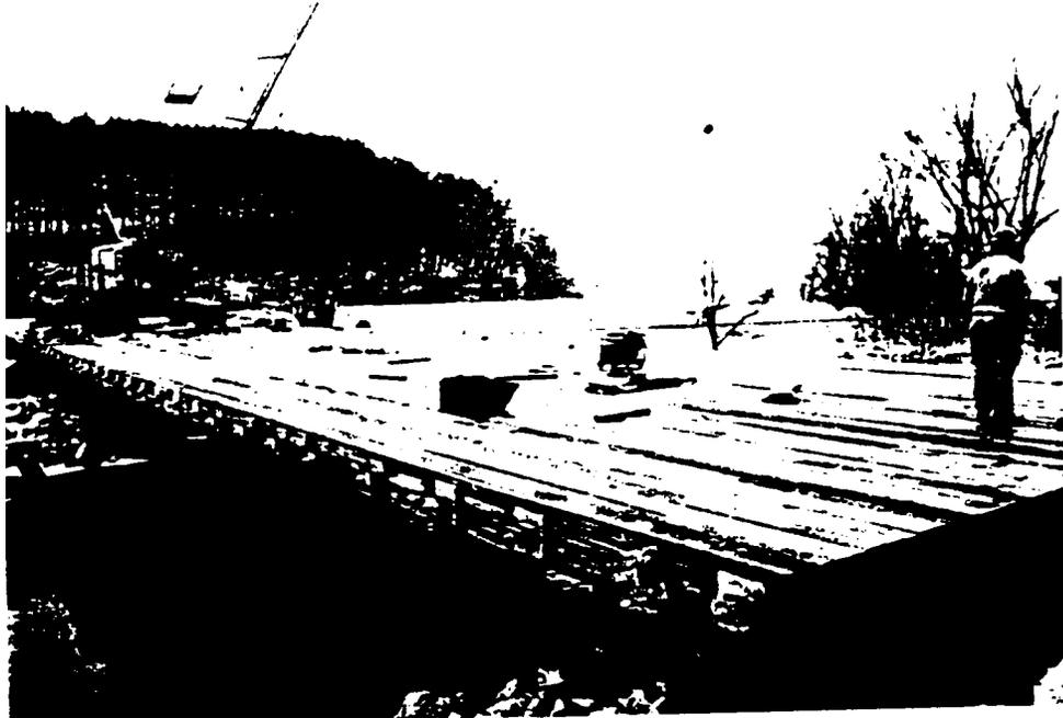
*Figure 12. The longitudinal glued-laminated timber deck of this timber bridge does not require stringers.*
