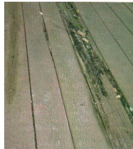
**All decks need regular maintenance.** Even cedar, redwood and pressure-treated lumber require regular application of a water-repellent preservative (including mildewcide). But lumber that is not naturally durable or that is not preservative-treated will quickly decay, resulting in a short-lived and vulnerable deck. Note the water intrusion around the long surface check of the leftmost deck board. In a year or two, this board will degrade to the same condition as the center board.
