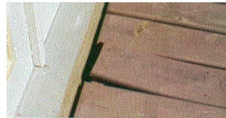
**Evenly dried, properly fastened boards resist warping.** Warping and cupping are usually caused by uneven shrinkage between the top surface and the bottom surface of wood. The wrong types or placement of fasteners also can cause wood to warp and cup, as shown above. Photo courtesy of the Southern Forest Products Association.
