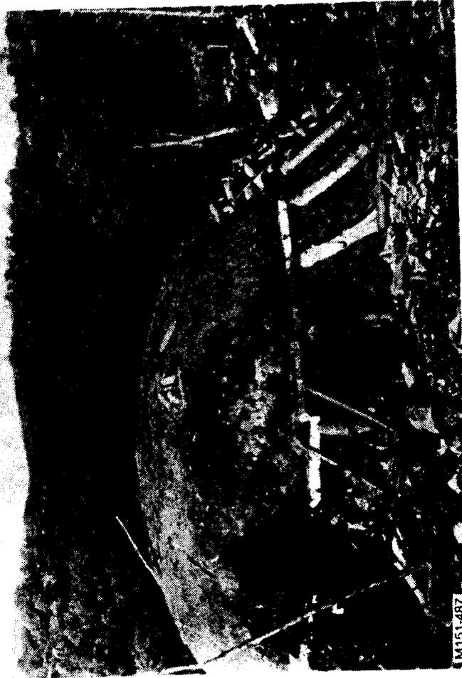
FIGURE 2 : Completed charcoal pit. Ladder is for climbing to the top to repair earth covering during cooling and to open the pit. Cross pieces keep earth from washing down during rains. Connecticut, 1901. (M151 487)
