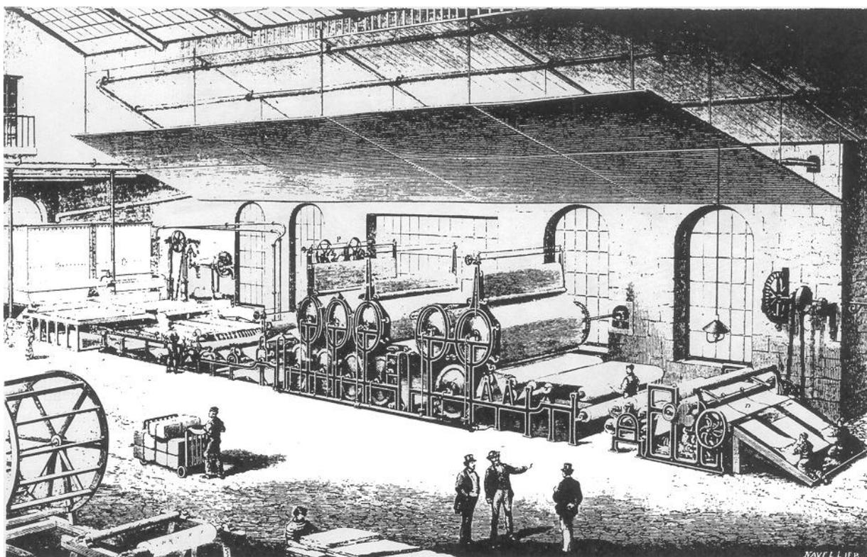
**Figure 5.** One of the first machines for continuous paper making, from wood pulp at left to cut sheets at right, was produced by Bertram and illustrated in Le Figuiier's *Les Merveilles de l'Industrie* in 1870. (Ann Ronan Picture Library.)
