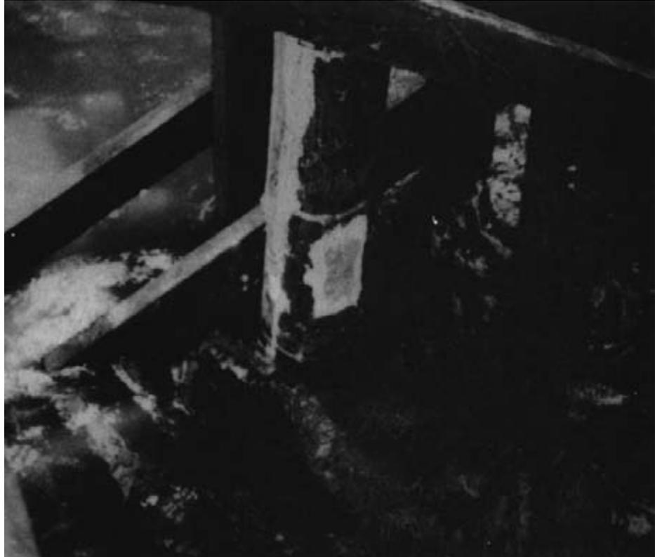
*Figure 14-15. - Epoxy gel surface repair of a timber pile (photo courtesy of Osrose Wood Preserving, Inc.).*
