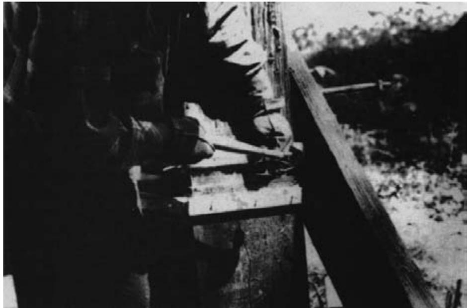
*Figure 14-18. - A joint for a post-injection epoxy repair is sealed with plastic wrap stapled to the members. Small wood strips are then nailed across the plastic to provide an additional seal (photo courtesy of Osmose Wood Preserving Inc.).*
