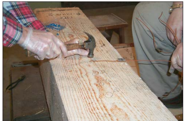
Figure 2—Toothpick being driven into 12- by 12-in. timber to seal thermocouple.
