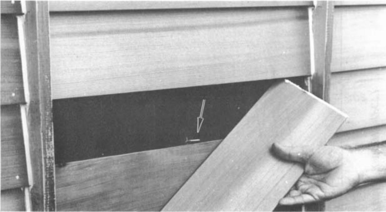
Figure 6. -- Moisture probe located immediately beneath siding
