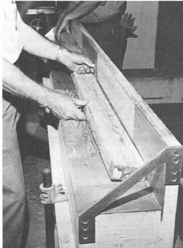
Figure 8.--Measuring bow in a stud.
