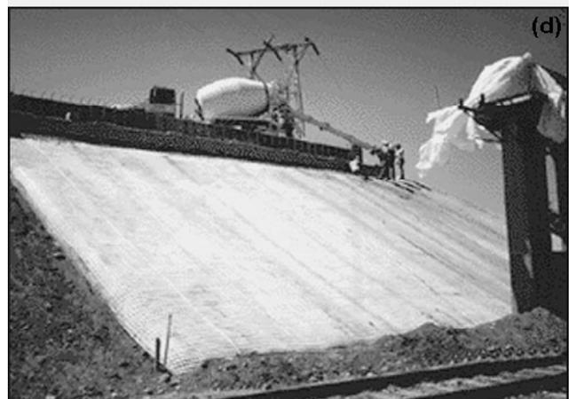
**Figure 5—(a) Filter point mat, (b) uniform section mat, (c) articulated block mat, (d) concrete mat being used on a slope. (Used by permission: copyright Elish Construction, Inc.)**
