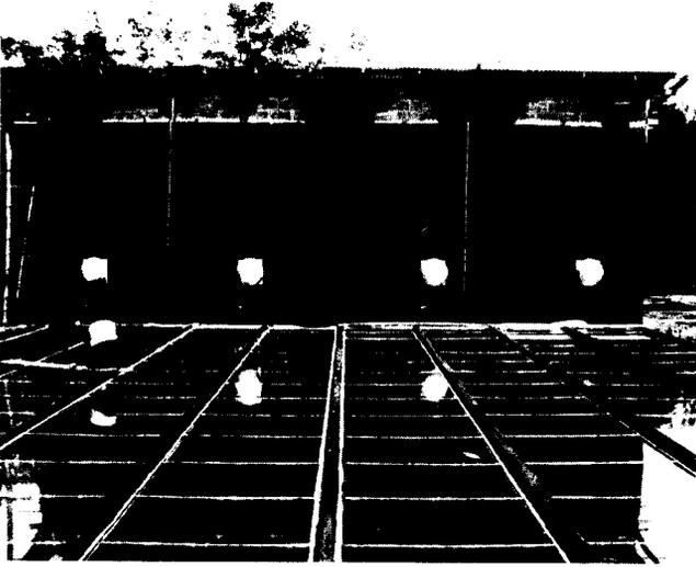
*Figure 3.—Partially completed 6,000 fbm solar/wood energy dry kiln at Borwood Ltd., near Colombo, Sri Lanka. (M84-0506-11)*
