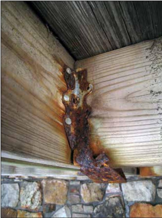
**Figure 2. Corrosion of a galvanized joist hanger and galvanized nails supporting a wood deck treated with a copper-containing wood preservative.**
