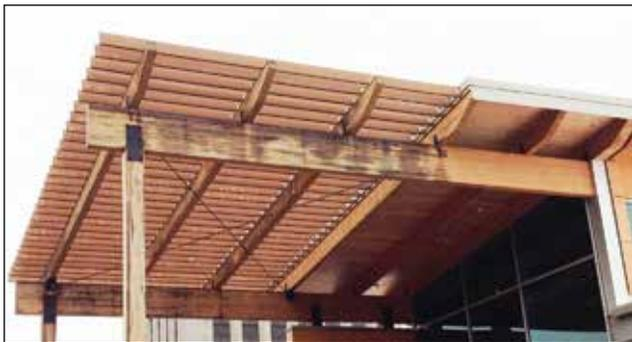
**Figure 10.** Illustration of the importance of roof overhangs for protecting wood from biodeterioration and corrosion. The right side of the beam is protected by the large roof overhang, whereas the left side is exposed to rain.
