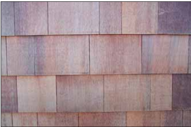
Figure 13. Shingles treated with tinted water-repellent preservative.
