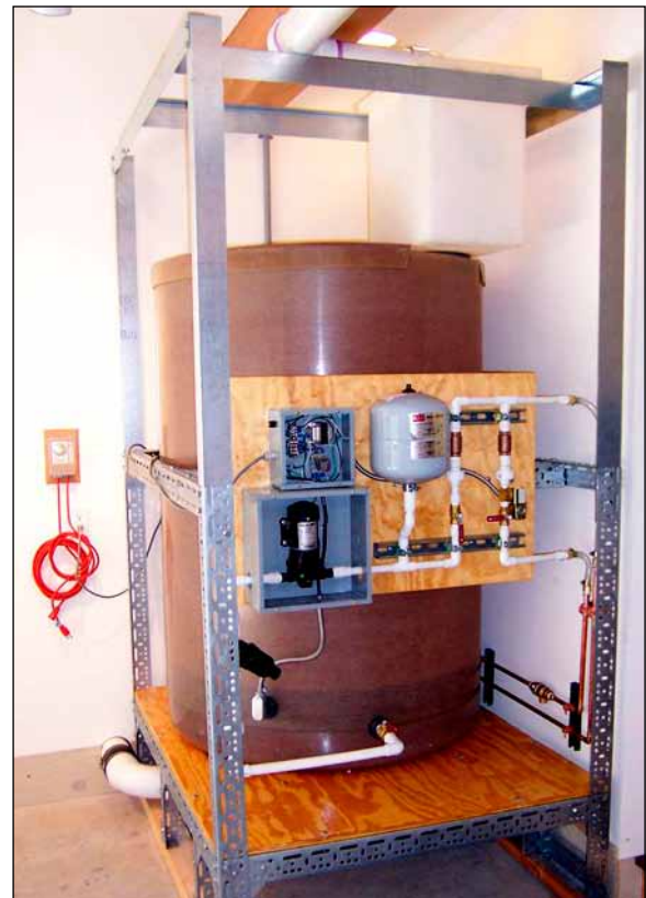
Figure 9. Non-potable rainwater storage and management systems for flushing toilets and washing clothes.
