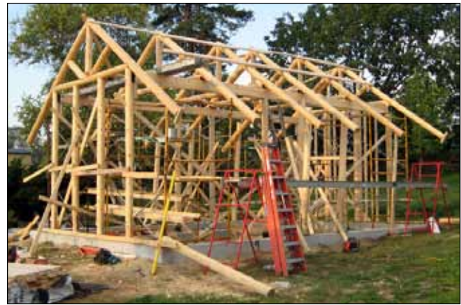
Figure 2. On-site structural assembly of small-diameter logs and trusses.
