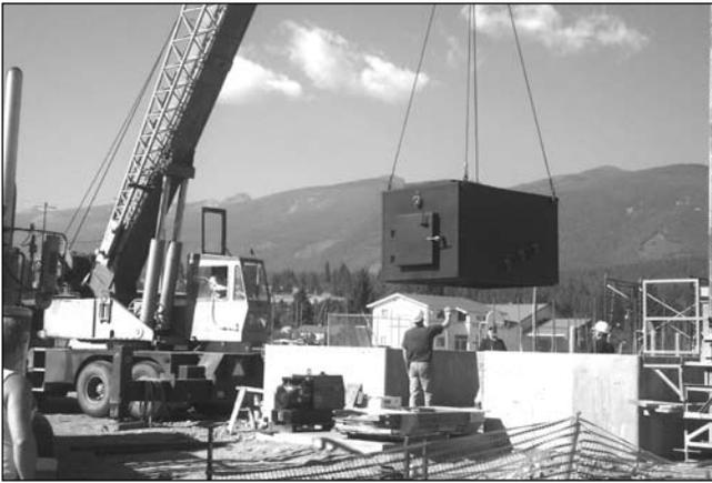
**Figure 3—Installation of wood boiler. Photo courtesy of Tim Maker, Biomass Energy Resource Center, Montpelier, Vermont. Used by permission.**
