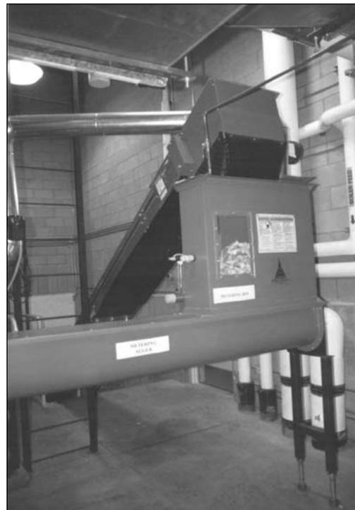
**Figure 6—Wood system fuel handling and metering bin. Photo courtesy of Tim Maker, Biomass Energy Resource Center, Montpelier, Vermont. Used by permission.**
