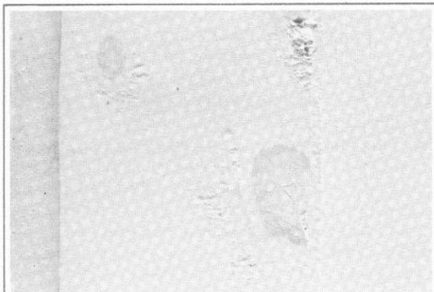
Figure 6. Brown discoloration of paint from resin exudation from a knot.
