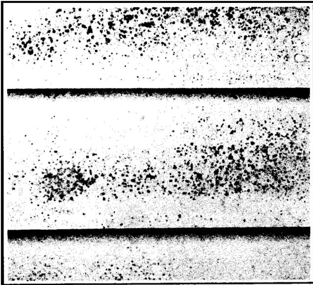
Figure 1. Mildew is most common in shaded or protected areas.
