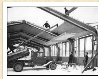
Glued-laminated (glulam) beams and arches use multiple layers of lower-grade wood to create large durable beams.
