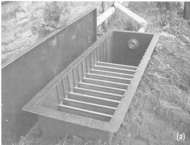
Figure 1. – Lignocellulosic filtration system: a) filtration box, b) filter frames inside filtration box.
