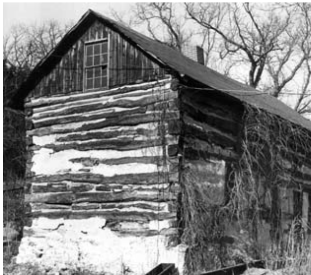
FIGURE 10.2 Old cabin built using solid wooden beams.
