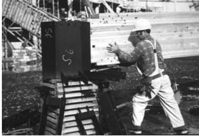
FIGURE 10.3 Large composite beam made from laminated lumber.
