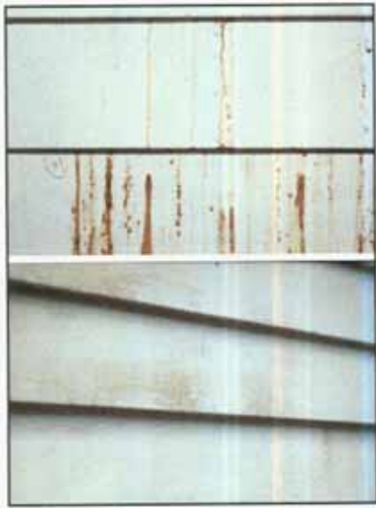
Figure 4—Examples of extractives bleed on finished wood.
