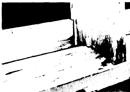
Photo left shows a window sash and frame treated with a water-repellent preservative and then painted. Photo right shows a window sash and frame that was not treated before painting. Both were weathered for five years. The painted on the treated surface is less weathered, the wood is in better condition, and the glazing is intact.
