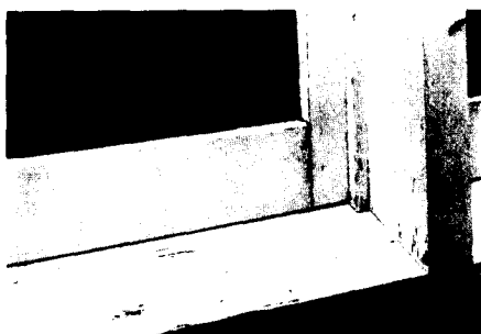
Photo left shows a window sash and frame treated with a water-repellent preservative and then painted. Photo right shows a window sash and frame that was not treated before painting. Both were weathered for five years. The painted on the treated surface is less weathered, the wood is in better condition, and the glazing is intact.
