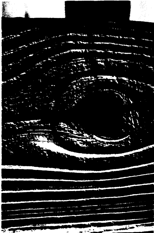
Note the weathered surface of this southern yellow pine after 20 years of exposure.
