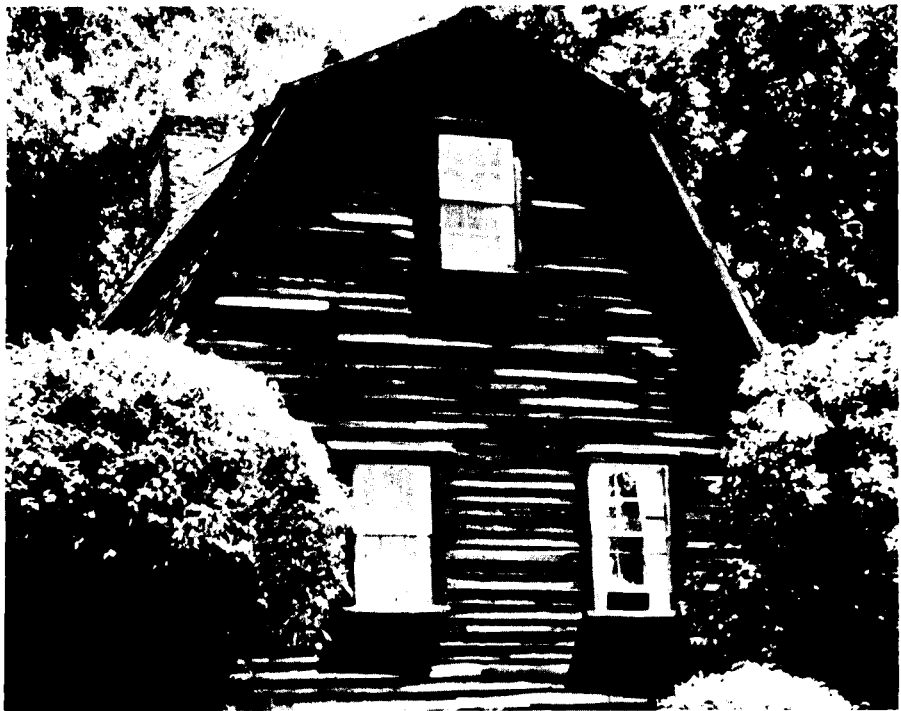
As an example of a Colonial "natural finish" house, the old Fairbanks House, Dedham, Massachusetts, was built in 1637. Most of the white pine clapboard siding was replaced in 1903, and has stood 80 years without paint.
