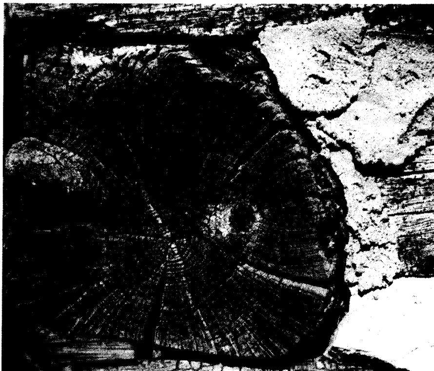
Figure 4. Close-up view of 140-Year-old weathered white oak logs of house shown in Figure 2.
