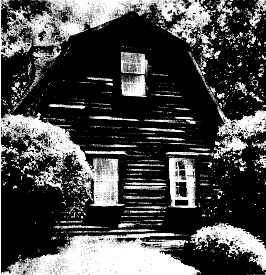
Figure 1. Old Fairbanks house at Dedham, MA, built in 1637. Most of the white pine clapboard siding was replaced in 1903, and it has withstood 85 years without paint..
