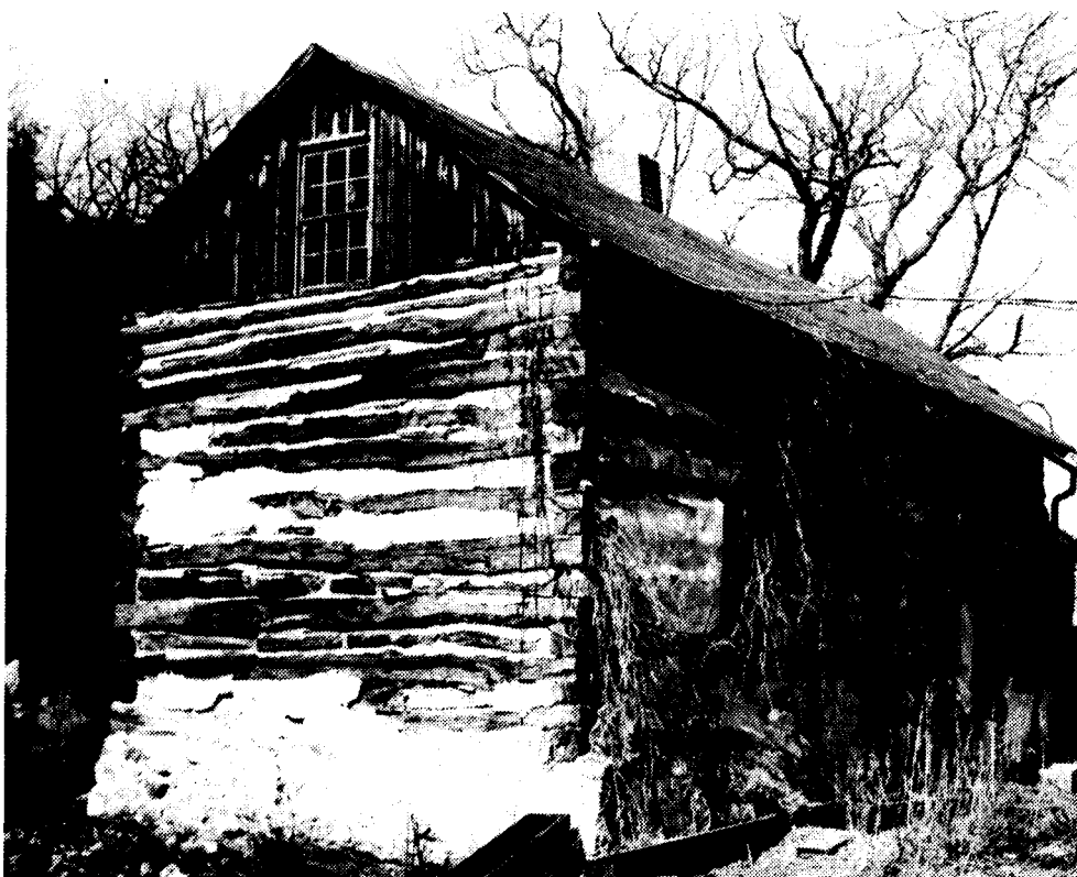
Figure 2. White oak log cabin near Middleton, WI, constructed around 1845 and never painted or finished.
