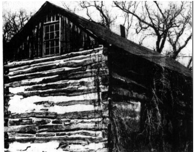
Figure 1.--White oak log cabin near Middleton, Wis., constructed around 1845 and never painted or finished.
