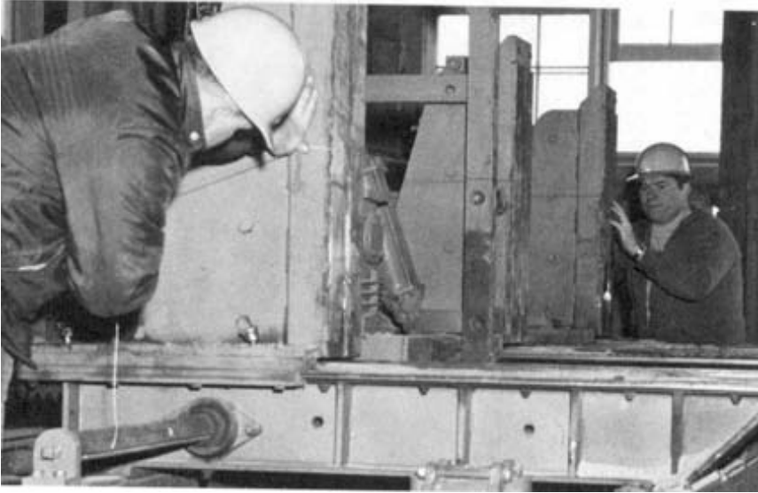
Figure 50. – Stretch a string across knee faces to check knee alignment.
