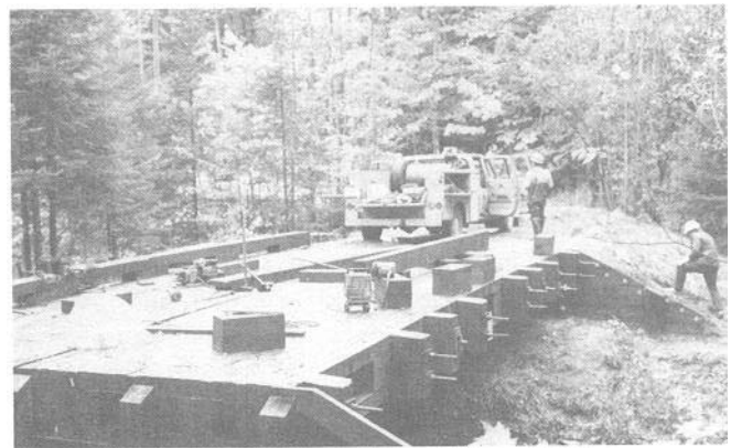
Figure 3—Bridge during construction—both panels in place. (M87 0288-4)
