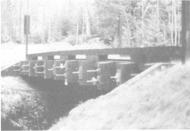
Figure 1—Mormon Creek Bridge.
