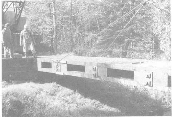
Figure 2—Bridge during construction—first panel in place. (M87 0280-18)
