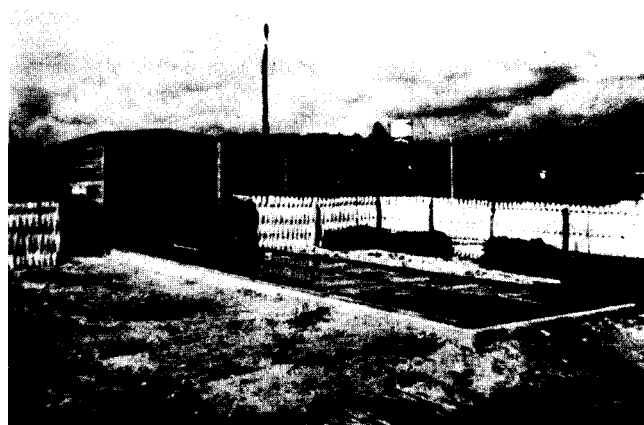
Figure 1.— 1,000-fbm (2.4-m 3 ) capacity solar kiln at Forest Research Institute, Yezin, Burma. (M152096-1)
